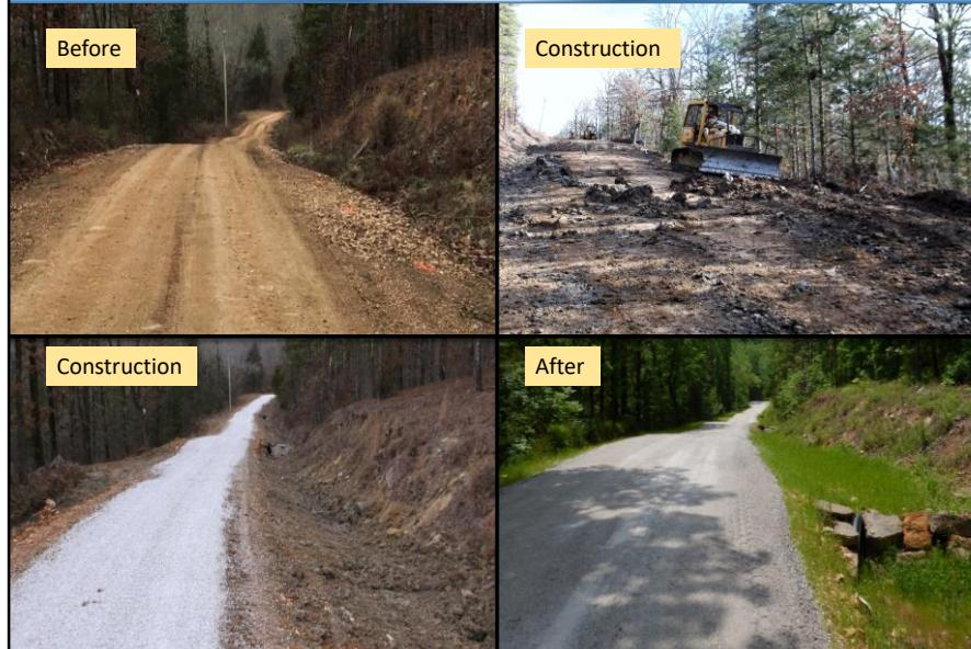
Meadow Creek Pilot Project as an example. Looks like a typical relatively steep, unpaved road when dry. Entrenched, Water flows directly over the road. Ditch is a direct conduit to the stream. Project consists of raising and building up the road bed, adding culverts, head walls so the culvert entrance doesn't erode, move the water out into the forest to be filtered before it gets to the stream. Add a driving surface aggregate that won't erode as much.
