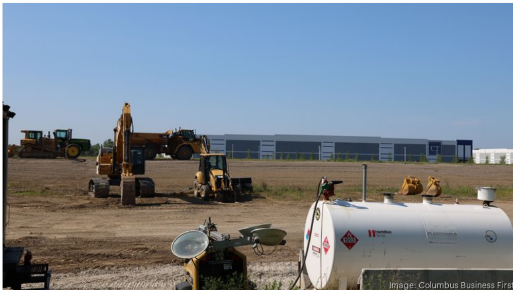
Construction equipment at the site of Anduril's campus in Central Ohio.
