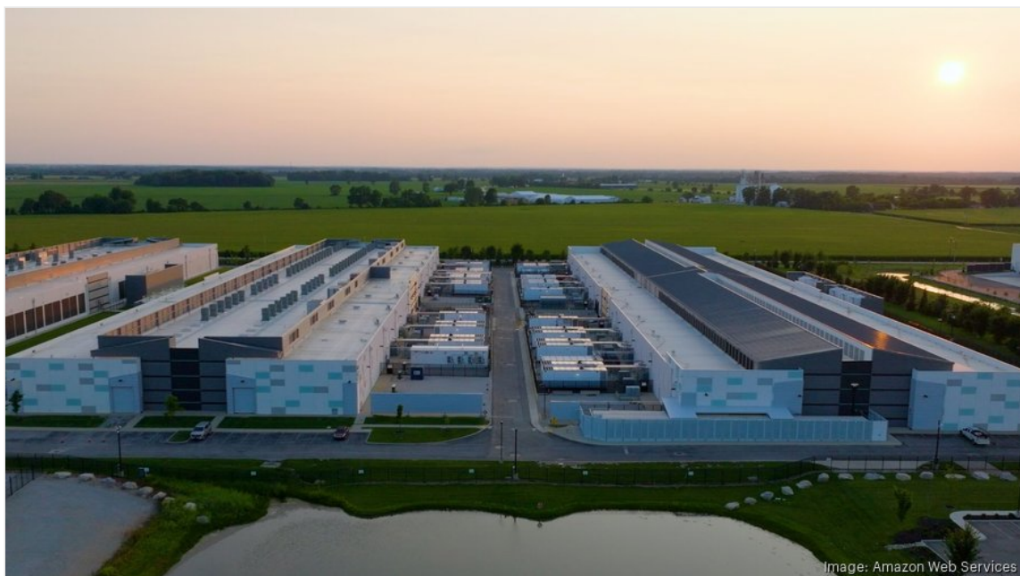
Amazon Web Services' data center campus in Dublin.
