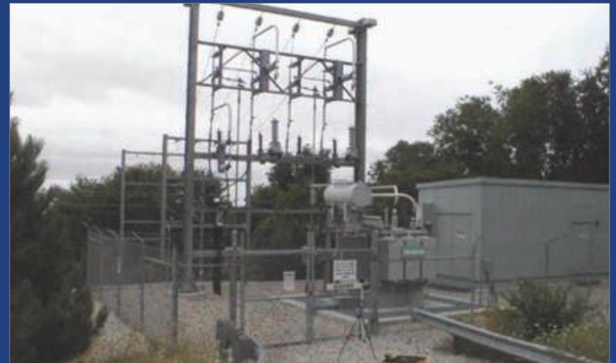
Example of Traction Power Paralleling Station
