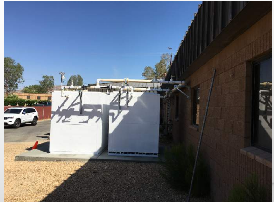
PhaseStor Install, rear service yard, B1020
