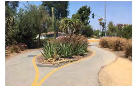
Example of diverter island that alert cyclists to upcoming intersection (Whittier Greenway Trail)
