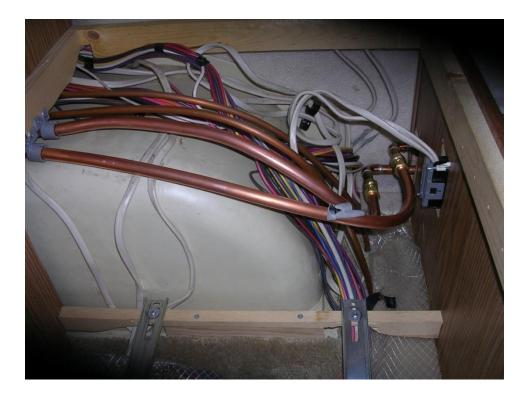
This picture is of the ½ inch flexible copper tubing carring hot water from the hot water tank and a return line to the tank. The other smaller lines are bringing water to the sink. Our hot water tank is to the left and on the other side of the refrigerator.
