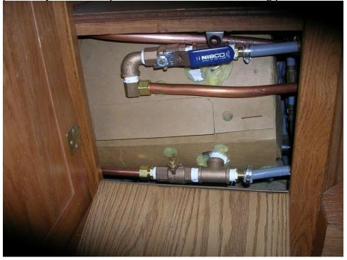
I started by installing tees and shutoff valves at the in and out ports on the hot water tank.
