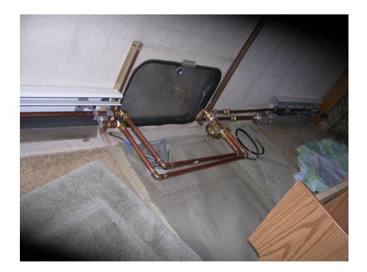
Under the forward seat of the dinette is the circulating pump. The rigid tubing follows the outer walls of the compartment that is assessable through the door, this compartment is under the forward seat of the dinette. To the right is another heat exchanger in the couch area.
