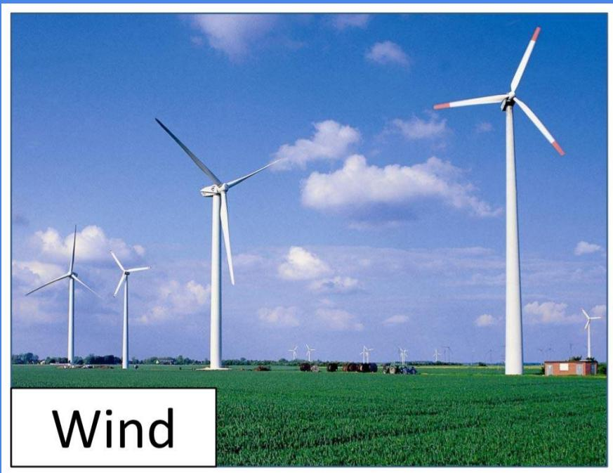
Wind can be used to create electricity, using wind turbines. As wind blows the blades on the turbine, they spin. The blades are connected to a drive shaft, which turns an electric generator to produce electricity.
