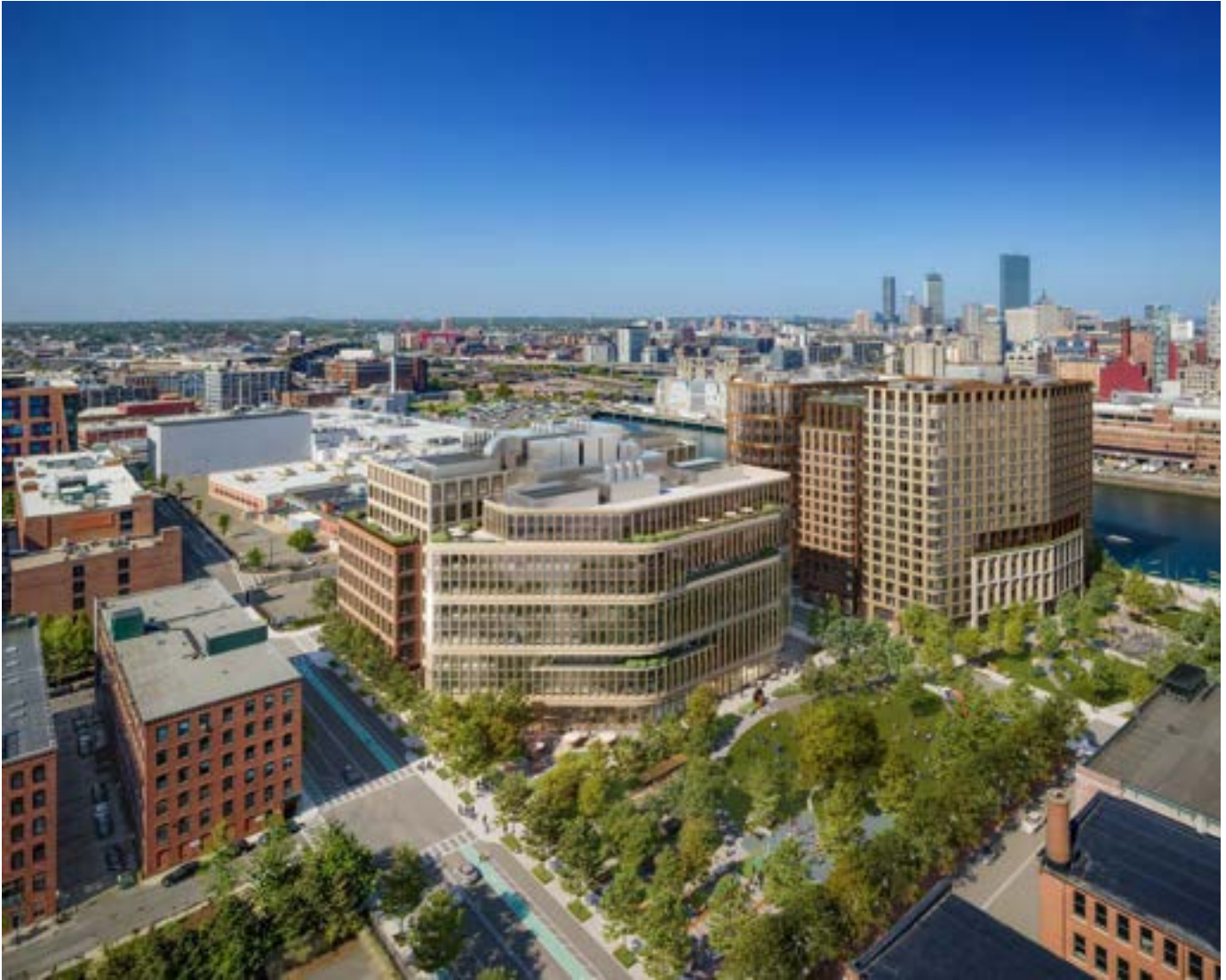
A rendering of the Channelside development planned for the Fort Point neighborhood of Boston. RELATED BEAL
