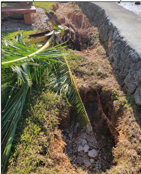
Figures 2 and 3: Erosion and undermining of the existing seawall built to protect the roadway is visible in within the study area. Photos courtesy of The Bureau of Statistics and Plans, Government of Guam
