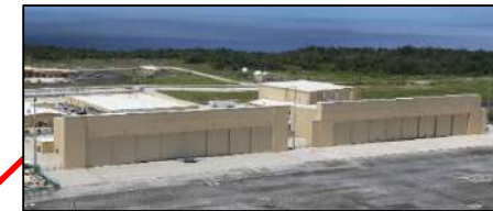
USMC North Ramp | Andersen AFB
