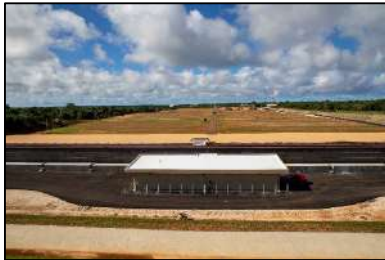
Mason Live Fire Training Range Complex
