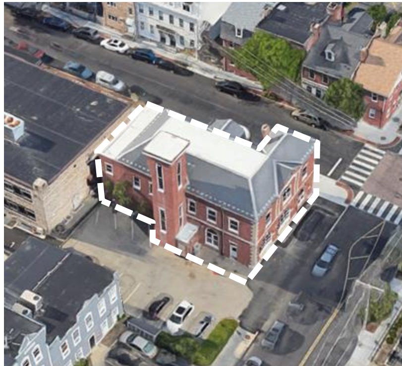
DPW ELECTRICAL (3 rd St)
