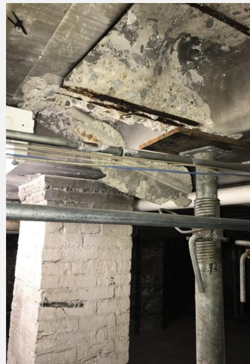
Lafayette Sq. Firehouse, critical improvements to address failing apparatus bay floor slab
