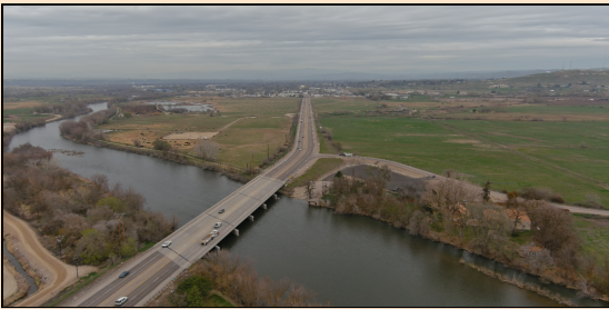
US-95 crossing the Payette River Bridge, facing north.
