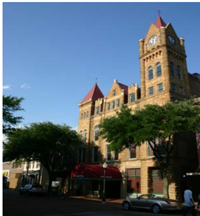
Sumter Opera House 21 N. Main Street Sumter, South Carolina
