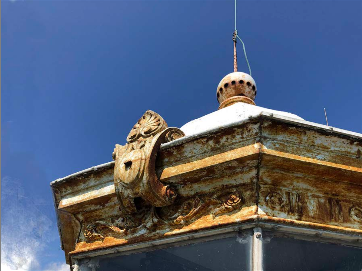
Photo 14. A cast iron cartouche, as well as embellishments of the lower fasciae, demonstrate the celebratory nature of Lighthouse design; these were the technological marvels of their time, expressed in architectural details such as these, as well as in literature and visual arts. Their allure is undiminished.
