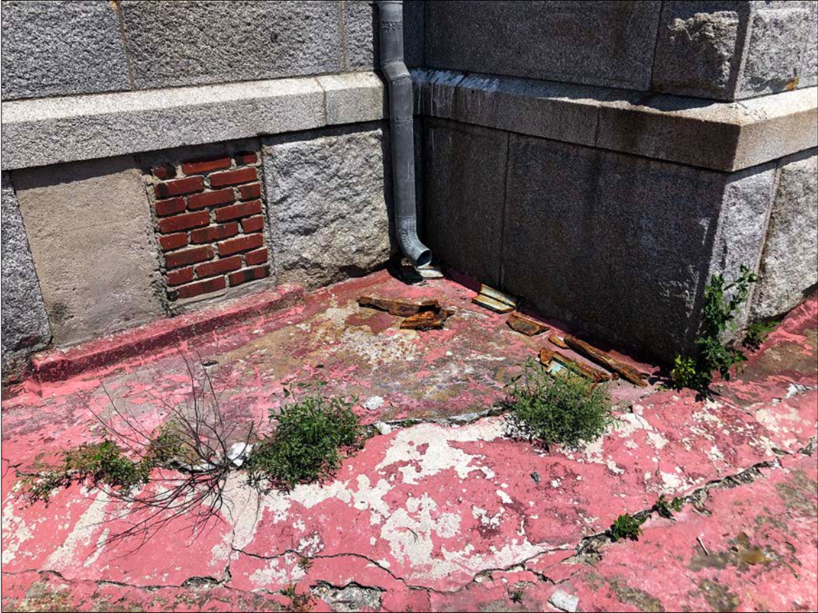
Photo 8. The Drum's deck surface is a crucial first line of defense, protecting the foundation and stores below. Cracks and breaching allow infiltration of vegetation and other organic matter, exacerbating the condition. Rainwater, left to spill adjacent to foundation walls, compounds deterioration. Note shards of cast iron that have fallen from the Lantern above.
