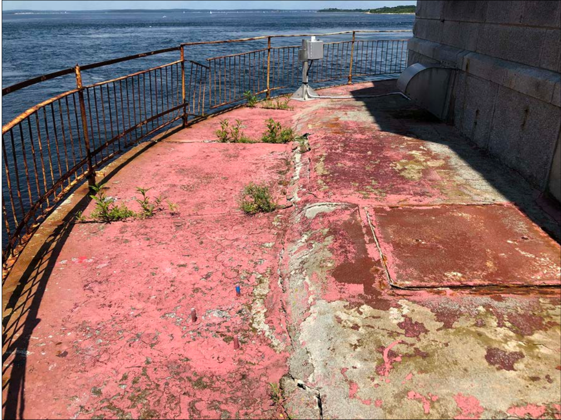
Photo 9. General view of the Drum deck and perimeter railing, both of which are currently in an unsafe condition. Bulkheads to the right provide access to the cellar and stores; in their deteriorated state, and without being safely cordoned, they harbor potential for a serious fall to nearly one story below.
