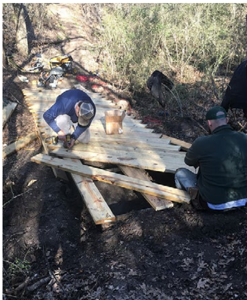
Garrett Fannin (left) and CJ Aitken attach deck boards to the first Canyon Ridge Trail bridge. FWNC&R Photo.
