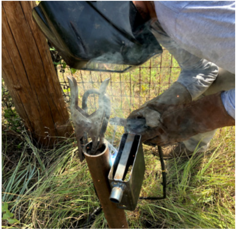
Nature Center staff welding the trail counter box to the pipe. FWNC&R Staff Photo.
