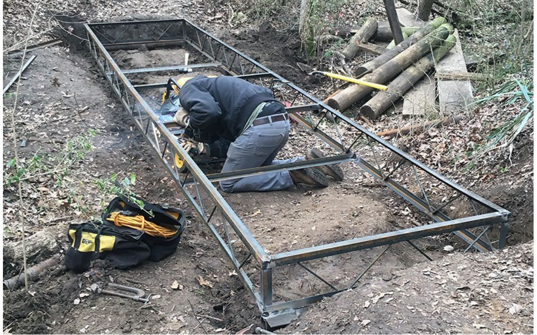
Welding the frame together for a new bridge on Canyon Ridge Trail. FWNC&R Staff Photo.
