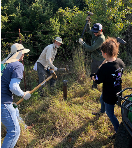
Driving pipe on which to mount trail counters is a team project. FWNC&R Staff Photo.
