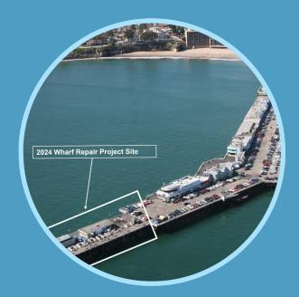
The project consists of the following elements: demolition of the Dolphin Restaurant and its associated enclosed patio; removal and disposal of damaged piles; installation/replacement of damaged or missing piles; and installation/replacement of associated structural members, mechanical connectors, and decking.
