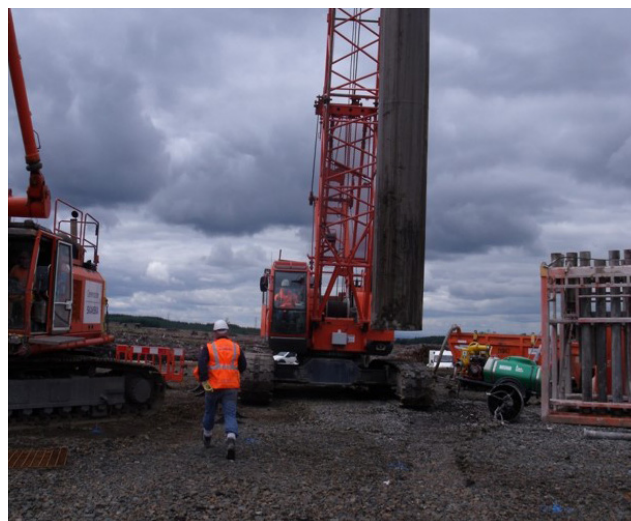
Spreading crane loads more widely enhances stability of the crane pad area.
