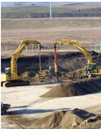
Rammed Aggregate Pier® Installation
