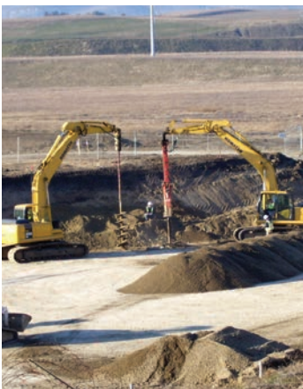
Rammed Aggregate Pier® Installation
