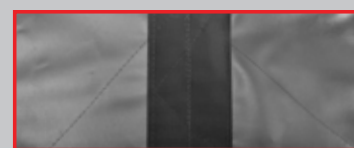
Patch over Seam
