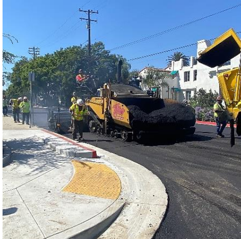
Example of Pavement Grind and Overlay and Access Ramp Construction on Castillo Street
