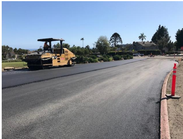
Pavement Grind and Overlay Construction Work
