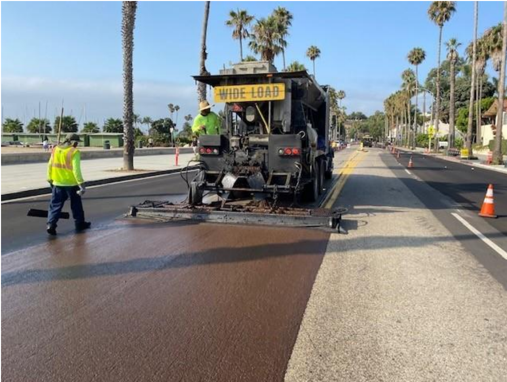
Slurry Seal Construction Work
