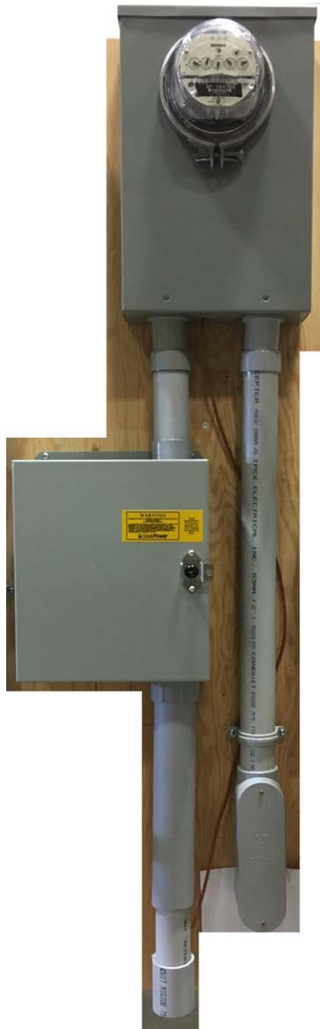
ESR Bulletin 2017-1 Figure 1: 200 A Self-contained Meter Socket Installation – Detail 1
