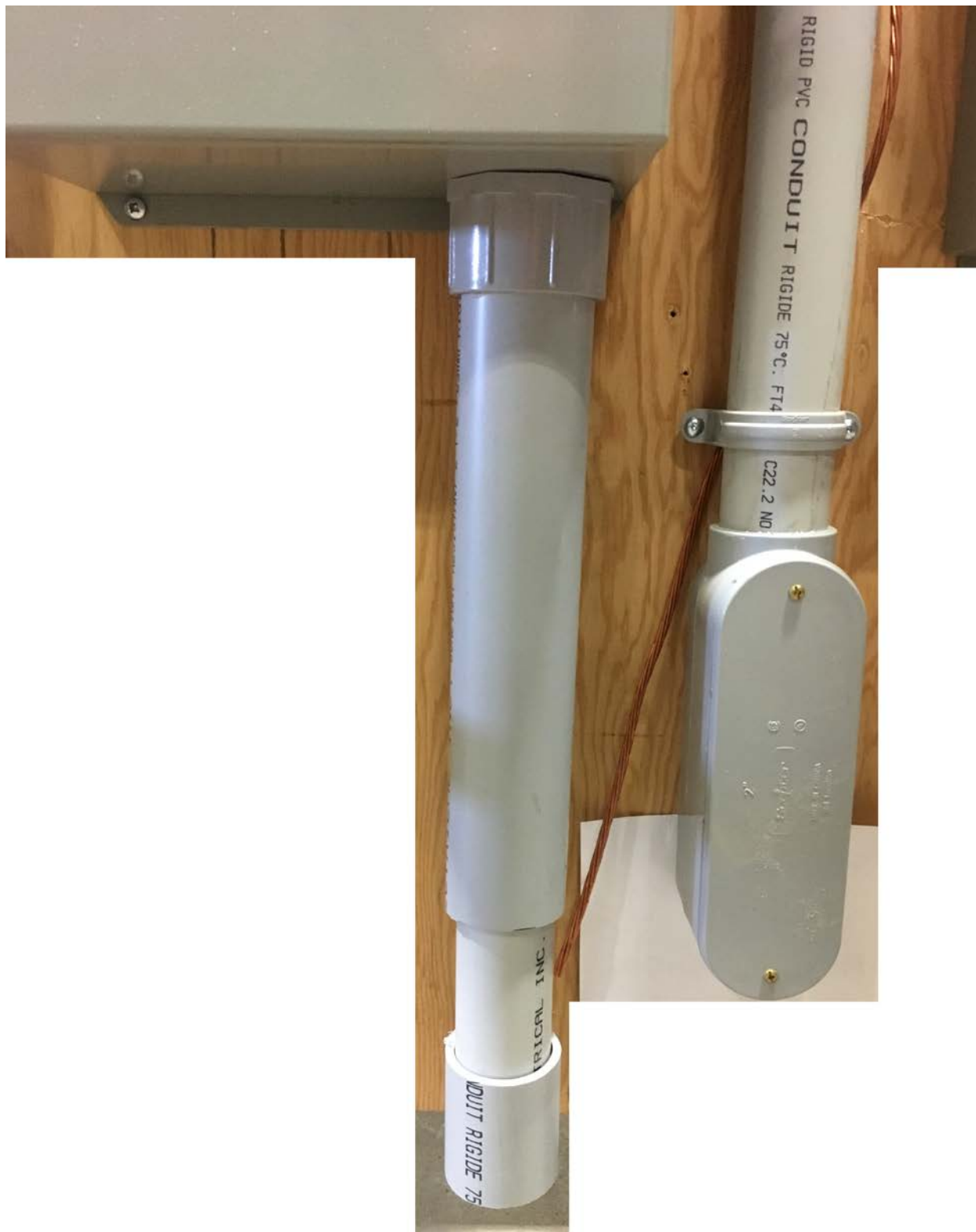
ESR Bulletin 2017-1 Figure 5: 200 A Self-contained Meter Socket Installation – Detail 5
