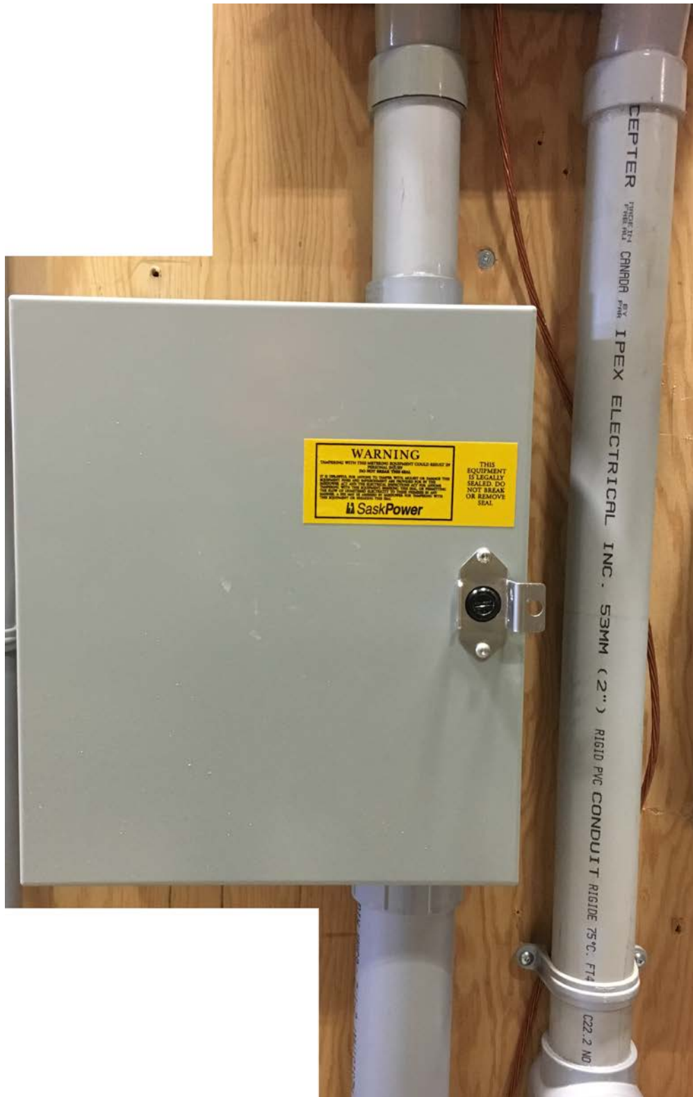
ESR Bulletin 2017-1 Figure 3: 200 A Self-contained Meter Socket Installation – Detail 3
