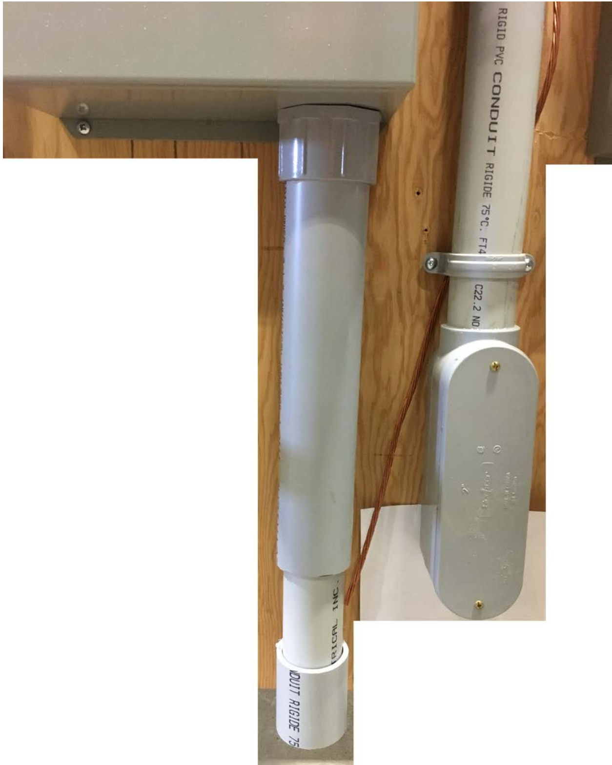
ESR Bulletin 2017-1 Figure 5: 200 A Self-contained Meter Socket Installation – Detail 5
