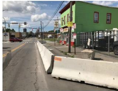
Concrete jersey barriers, min. 32" high
