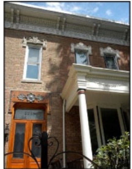
Shared wooden cornice runs along roofline
