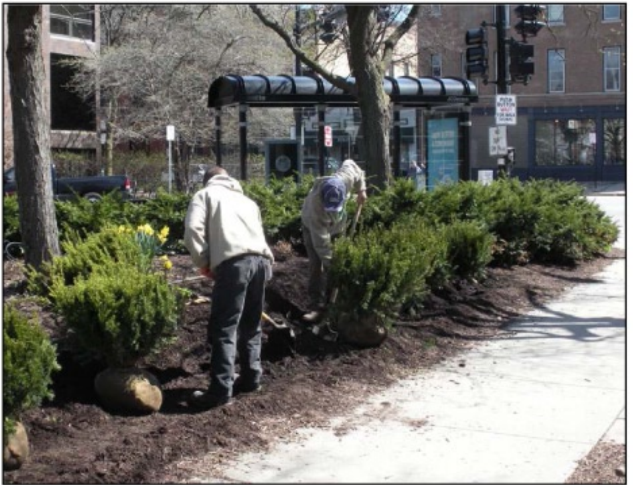
15 large evergreens being installed along the sidewalks
