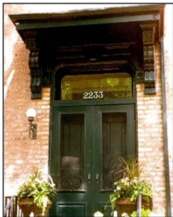
Pent style porch roof
