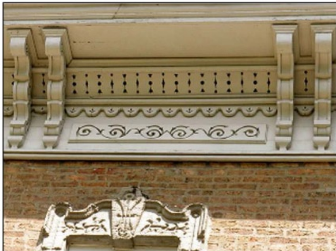
Closeup of cornice
