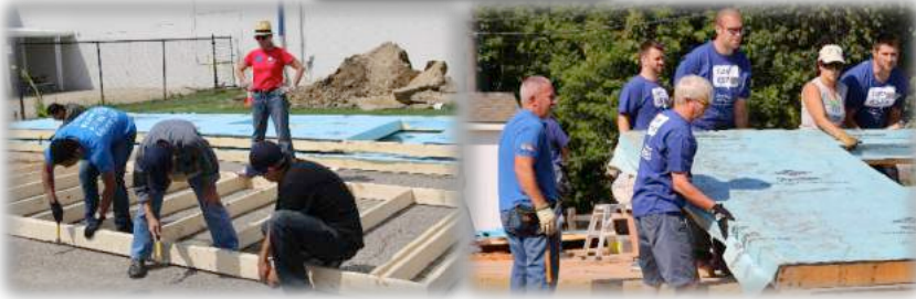
Walls assembled in then KSPG's parking lot, then brought to site...
