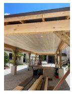
Finished trim around the columns is expected to be delivered soon. Then they will finish the trim for the rest of the beams, all the columns, and braces. Painting and trim out electrical will follow. The end of July is the current projected date for completion!
