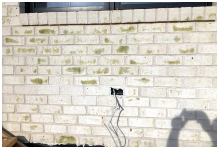
Figure 1 – Example of Vanadium Staining
