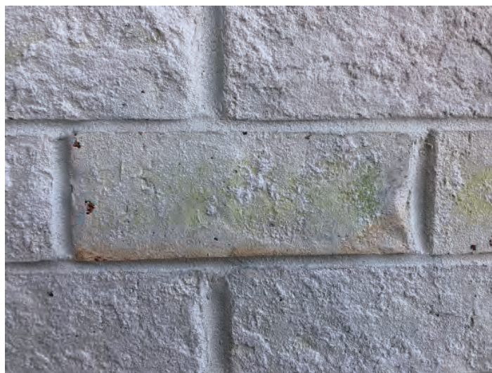
Figure 2 – Efflorescence/Staining Cycle
