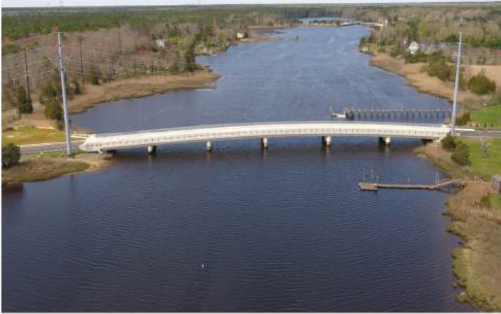
Replacement of Nacote Creek Bridge (PR-07), Old New York Road (CR610) over Nacote Creek, Owner: Atlantic County, Designer: Michael Baker International, Contractor: South State, Inc.
