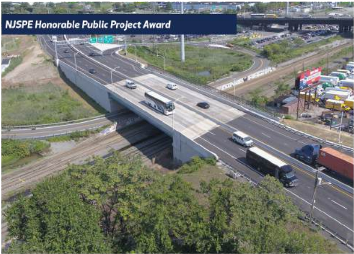
Route 3, Bridge over Northern Secondary and Ramp A, Owner: NJDOT, Designer: Michael Baker International, Contractor: Ritacco Construction, Inc.
