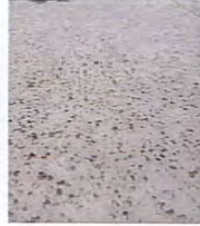
CIP CONCRETE PAVING - SALT ROCK FINISH 32-13-13A
