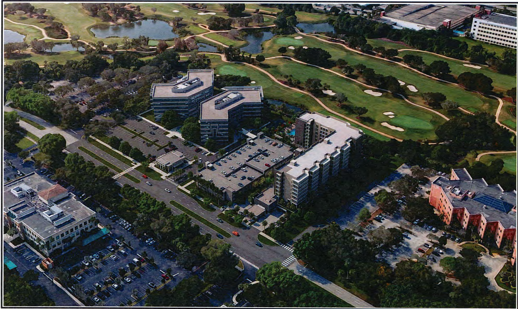
AERIAL VIEW - NORTH EAST
