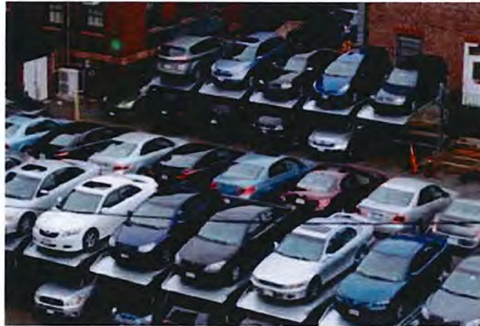
Above: Typical tandem installation without set backs, architectural screening or fire sprinklers.
