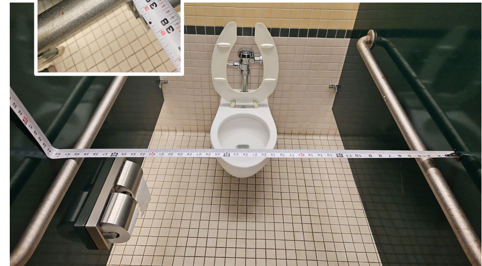
Accessible restroom lacks dimensions at Topstone Park
