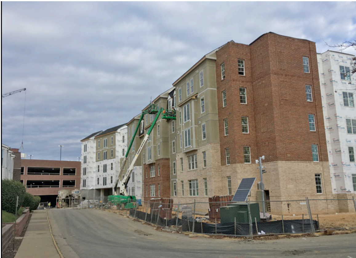
Windows in and the facade going into place.
