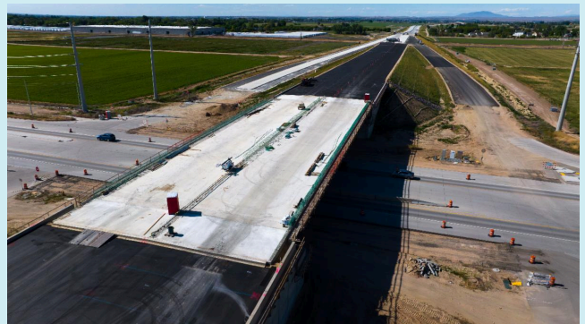
Franklin Rd: Recent concrete work on top of bridge and paving work on ramp approaches.
