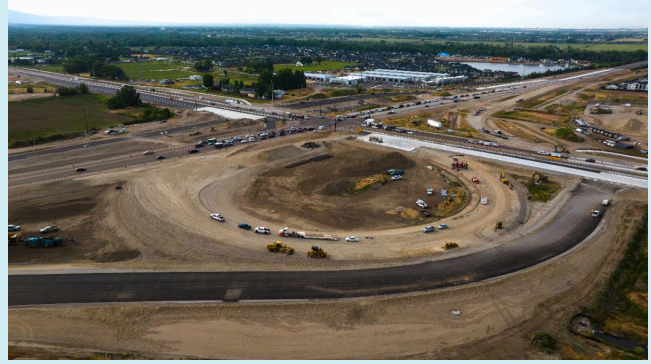
SH-44: Earthwork to form the base of the SH-44/SH-16 loop ramp.
