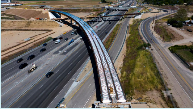
I-84: Flyover ramps on I-84 and recent work on ramp bridge decks (top of bridge).
