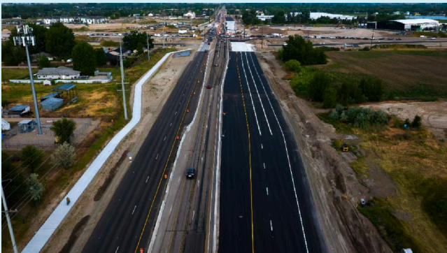
SH-44: Recent pavement work along the northside of SH-44 looking west toward SH-16.
