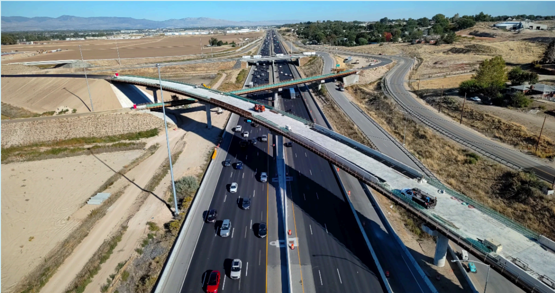
Flyover ramps over I-84 looking east.
