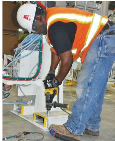
LEFT: Millwrights are installing all processing equipment, including conveyor systems and robots that will paint and weld body panels.
