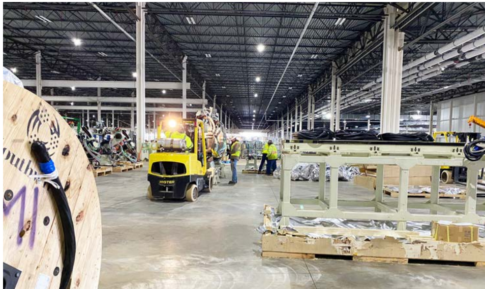
LEFT: Millwrights are installing all processing equipment, including conveyor systems and robots that will paint and weld body panels.
