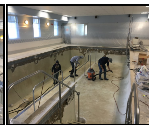
Old plaster and tile out
