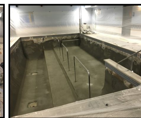
Rough plaster first layer
