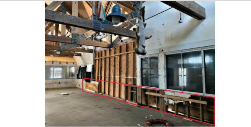
INTERIOR - SALES ROOM / MAIN ROOM: Locations of Painted Wood Built-In Cabinetry with Drawers, Destroyed by Storm Debris
