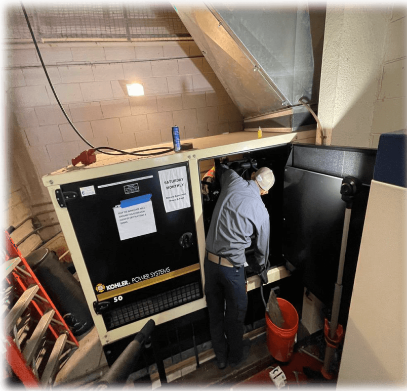
Fire Station Generator Inspection
