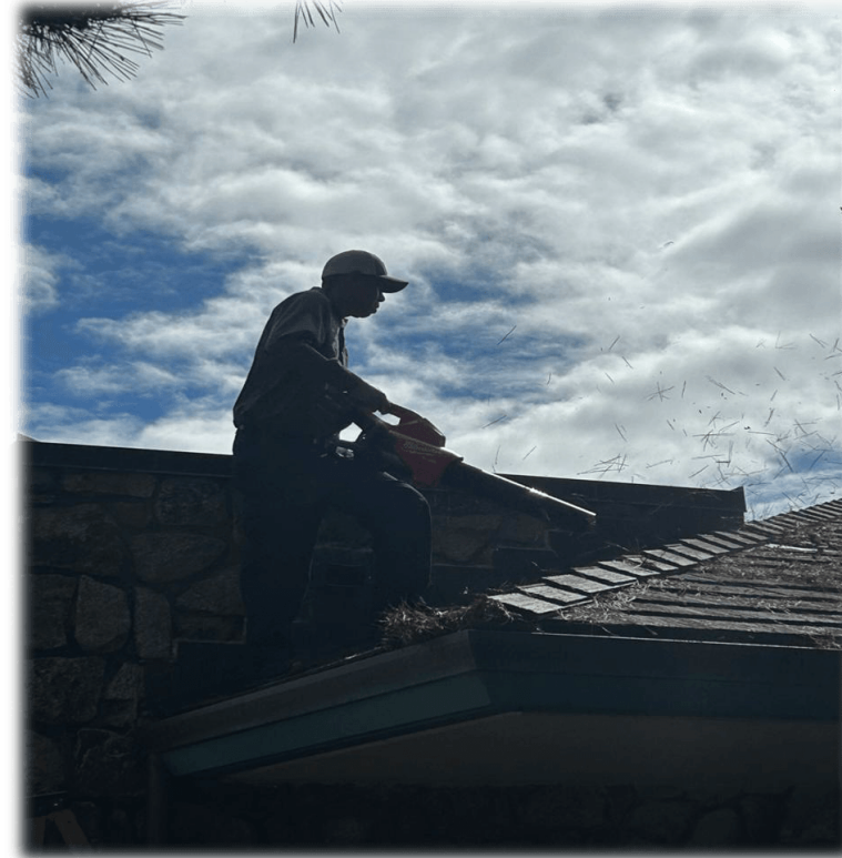
Children's Library Roof and Drainage Cleaning
