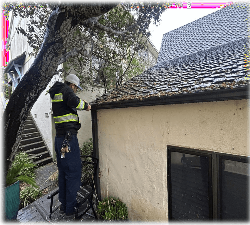
City Hall Gutter Repair
