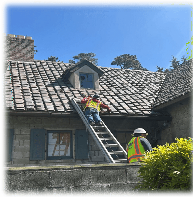
Flanders Mansion Leaky Roof Repair
