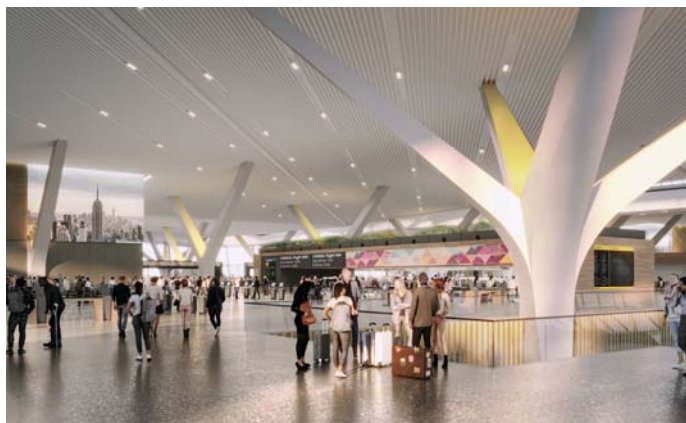
The New Terminal One at JFK will feature 26 sculptural tree columns to anchor the terminal's "butterfly roof" structure. Modeled on the aerodynamic flow of air, the structure was built to evoke the feeling of flight and are said to embody the core values of elevated architecture, thoughtful design, and an inspiring sense of place.
