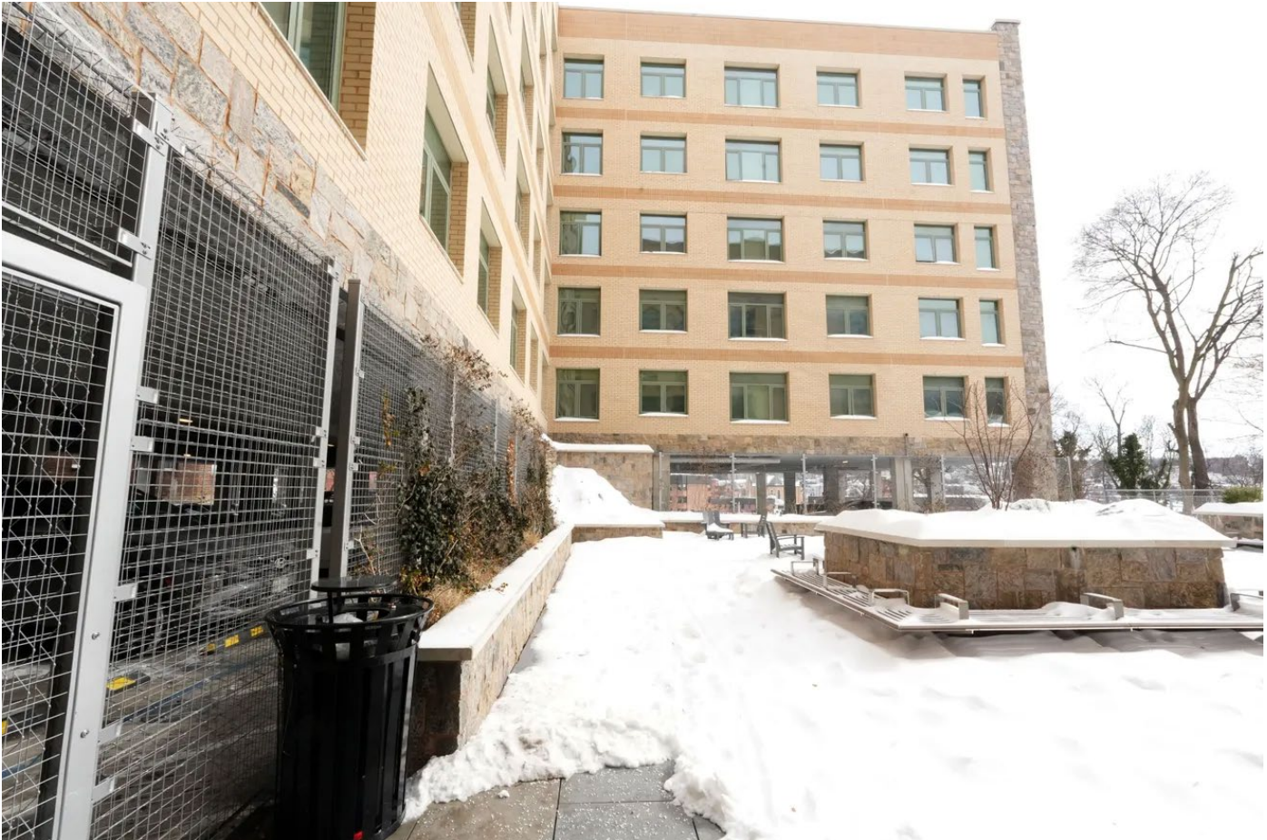
The Summit on Hudson, a 113-unit affordable housing eco-friendly residence in Yonkers Jan. 27, 2026. The Westhab building has designated 45 units to supportive housing for residents transitioning from shelters. Tania Savayan/The Journal News
