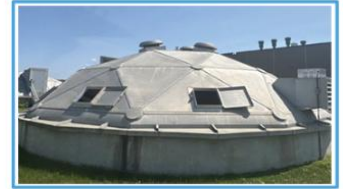
Jordan Water Treatment Facility
