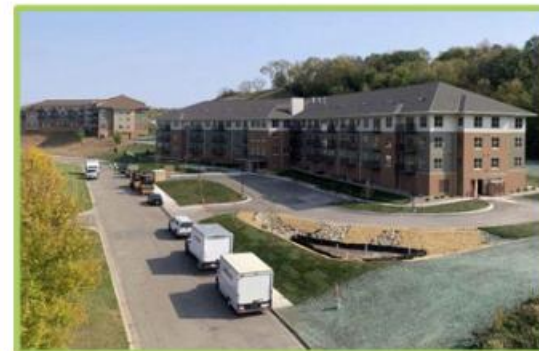
Housing project in Scott County
