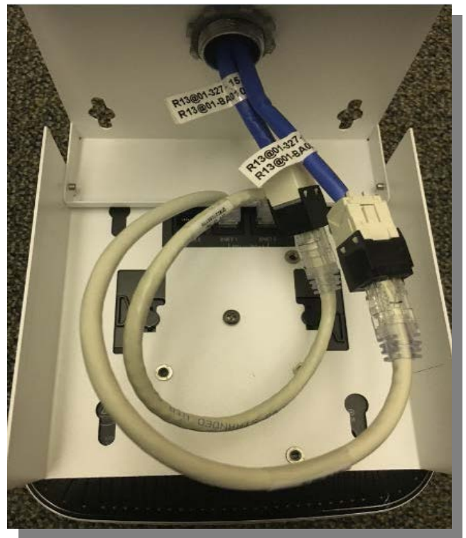
Model 900-HC Pendant or "Hanging Conduit" mount is a larger box than a standard junction box, permitting convenient concealment of cable termination and patch cord.
