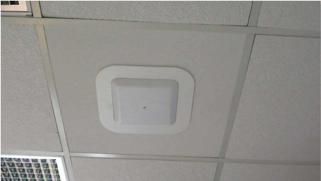
Model 1044-CCOAP3800 Recess AP Installation Kit for 2' x 2' Suspended Ceiling Panel with Cisco 3800 Series AP
