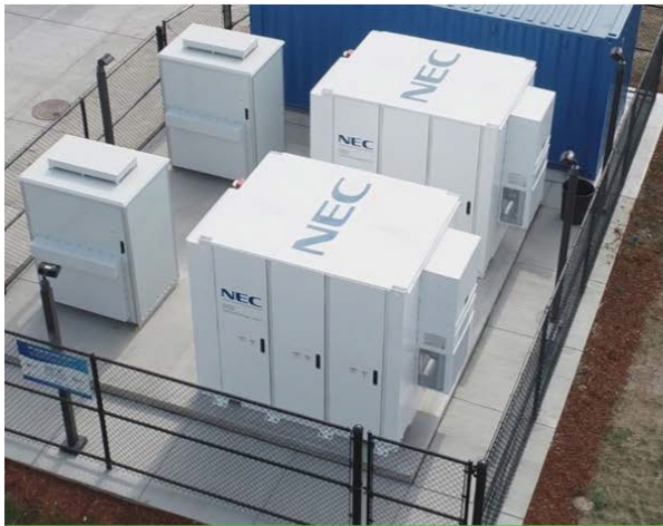
Battery Energy Storage System
